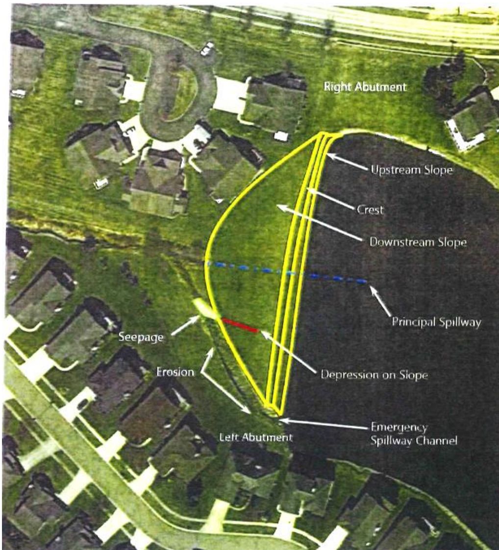
Figure 1 – Existing Dam Features Source: ODNR Dam Safety Inspection Report Nov. 25, 2019
