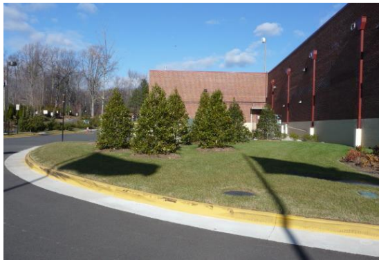
Figure 1111-C: The above image illustrates a vegetative screen that hides HVAC equipment and a dumpster.
