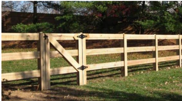
Figure 1109-C: Example of where wire fencing has been mounted on the interior of an approved three-rail fence.
