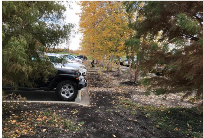
Figure 1111-B: The above is an image of a stormwater infiltration island used in a parking area.
