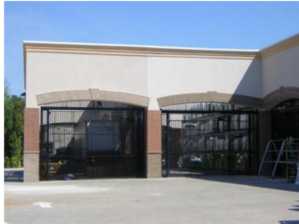
Figure 1111-D: The above image illustrates a wall and fence that is an extension of the principal building that is designed to screen outdoor storage areas.
