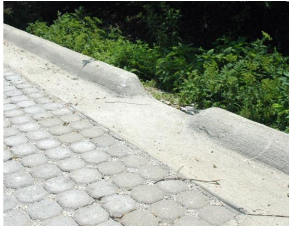
Figure 1112-A: Cuts in the continuous curb allow for stormwater to be directed into landscaped areas.
